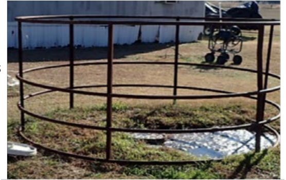
Photo-1: A failing OSSF site.
